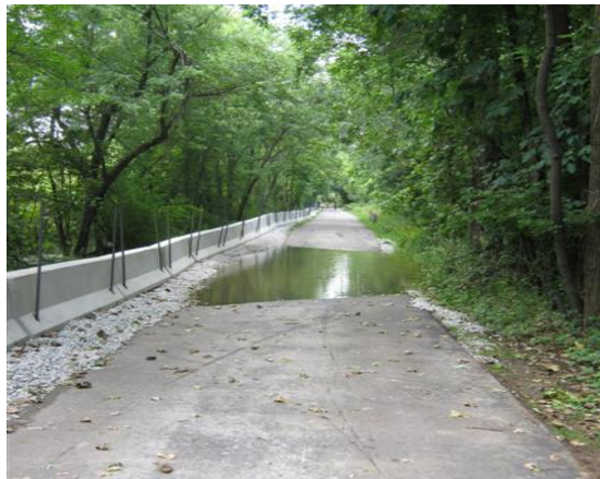
Completed concrete barriers prevented overtopping in the July 24-25 flood event of 2010 along the Des Plaines River.
